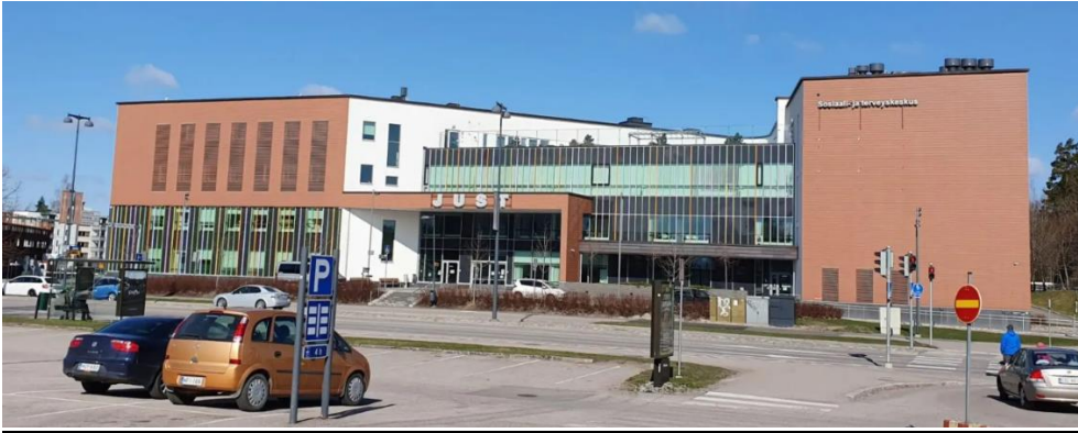
Fig. 27. Social and health care centre in Järvenpää. Photo. Rototec Oy.
