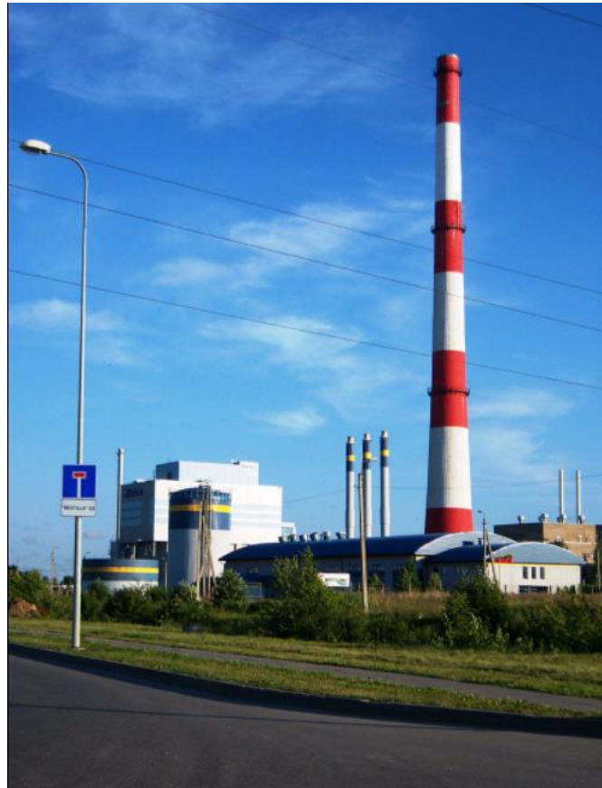
Fig. 39. Klaipėda geothermal demonstration plant. Photo: https://en.wikipedia.org/wiki/Klaip%C4%97da_Geothermal_Demonstration_Plant
