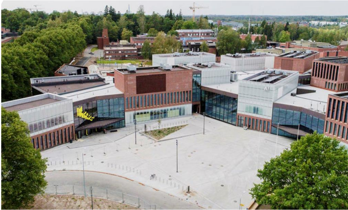
Fig. 26. Aalto University's new campus block in Otaniemi, Espoo heats and cools with geoenergy. In the building there is also a small shopping centre and entrance to the metro station. The energy well field was mainly implemented under the building next to the metro tunnel. Photo © Aalto University / Mikko Raskinen.
